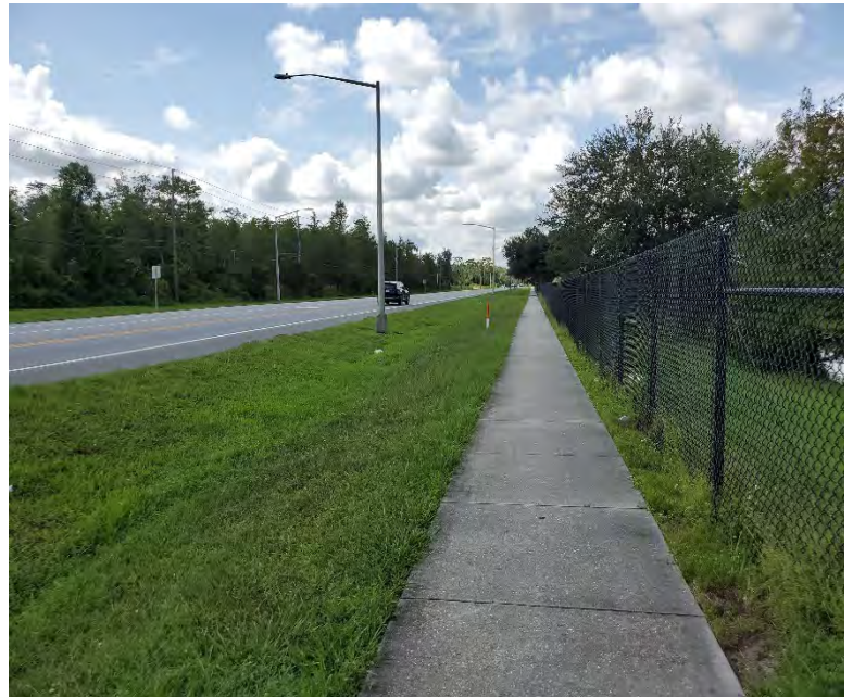
Roadside ditch facing south
