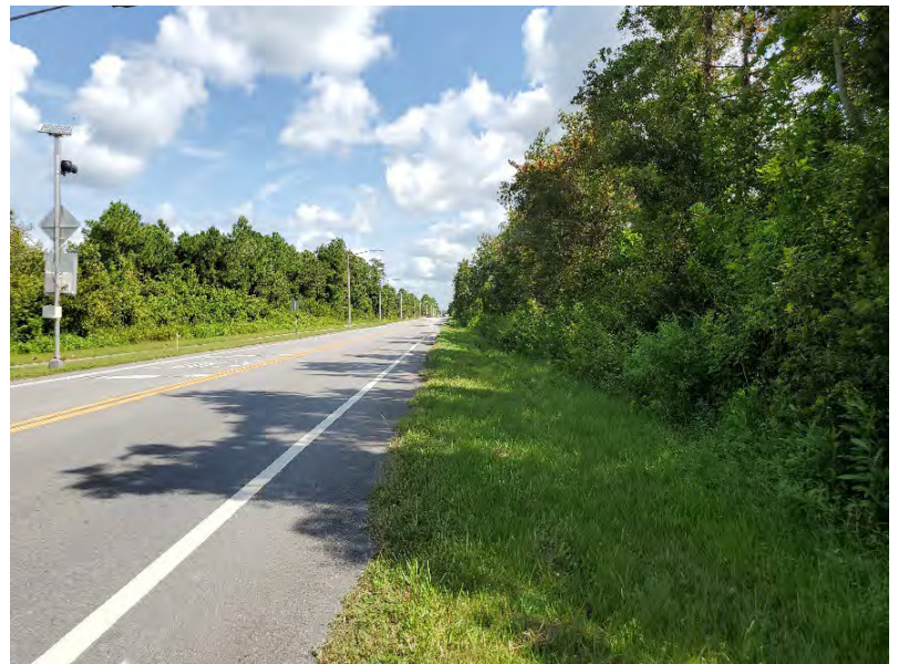
Roadside ditch facing north
