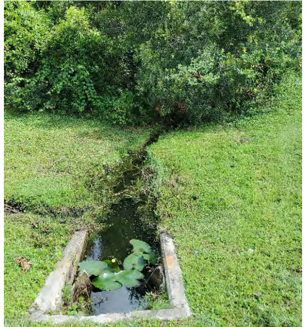
Existing side drain under Corner Lake Drive which conveys runoff from Basin 2B to Basin 3
