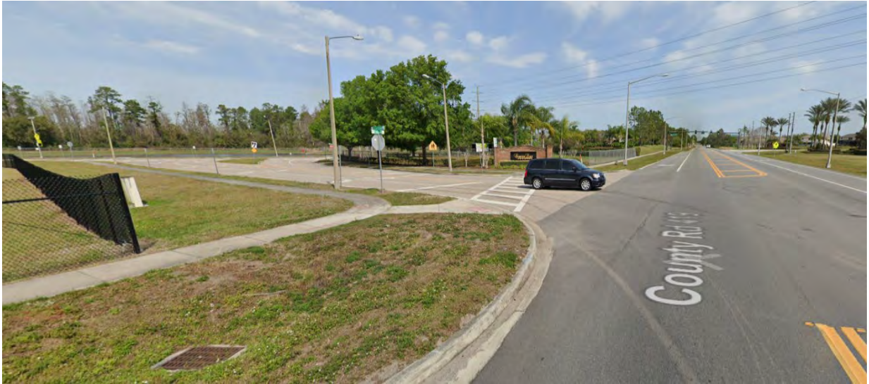
Chuluota Road and Schoolview Way showing ditch bottom inlet which drains to existing pond
