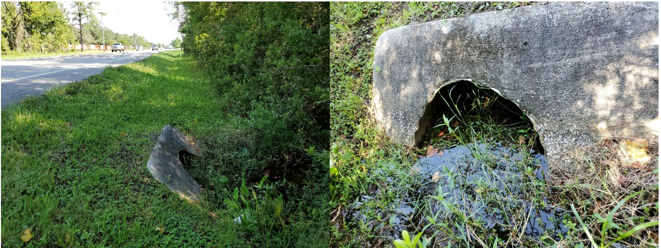
Existing cross drain (east side)
