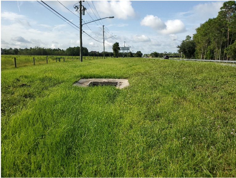
Ditch bottom inlet which conveys sheet flow from Chuluota Road to existing storm drain, facing south.
