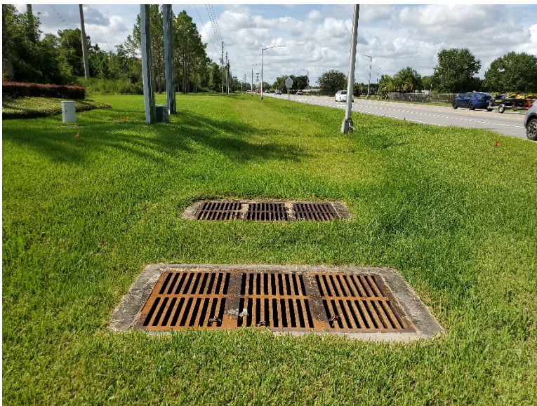
Roadside ditch facing south. These inlets convey runoff under Cypress Lake Glen Blvd.
