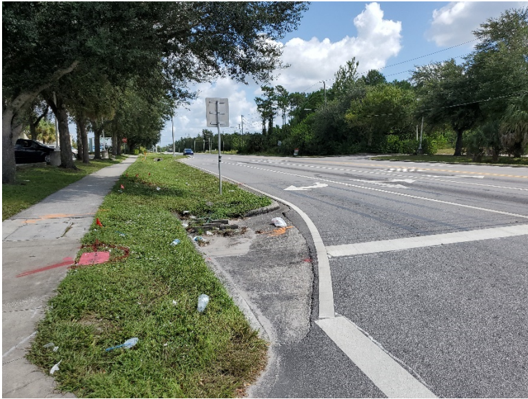
Existing inlet which drains west in FDOT SR-50 storm drain. Photo facing north.
