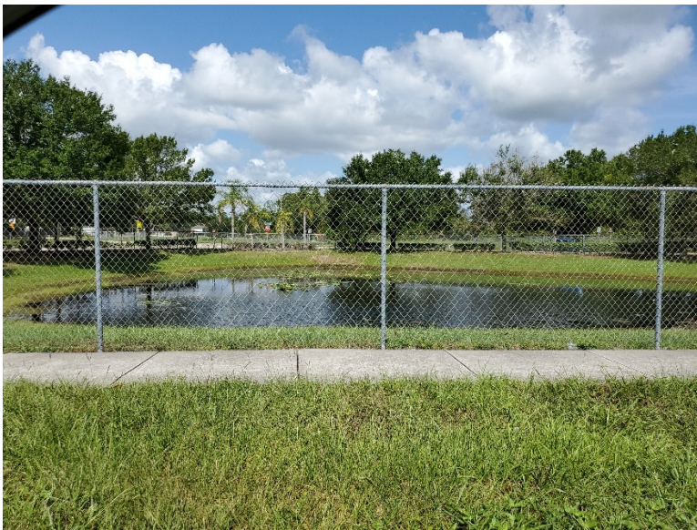
Existing pond on Schoolview Way
