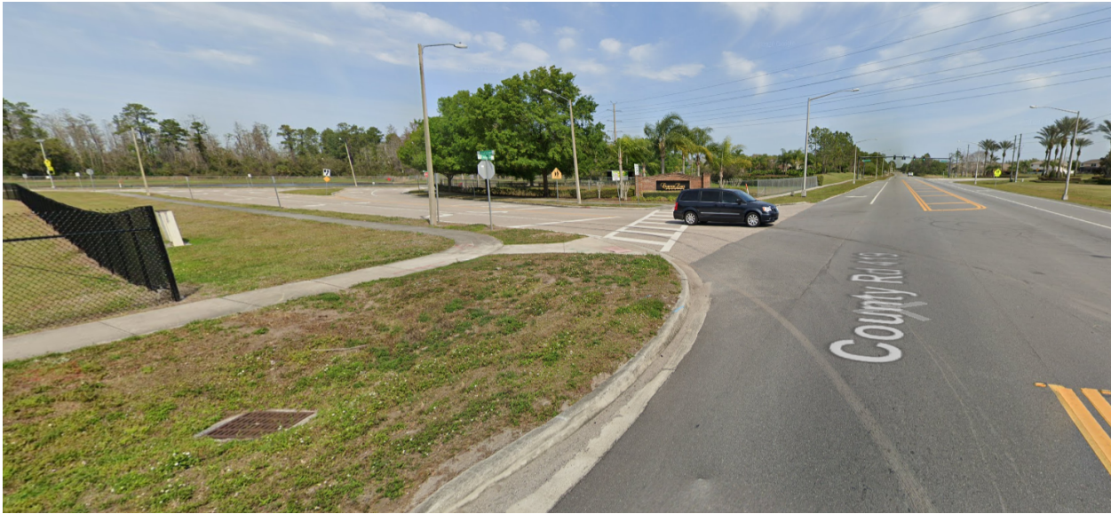
Google Street View of Chuluota Road and Schoolview Way showing ditch bottom inlet which drains to existing pond.
