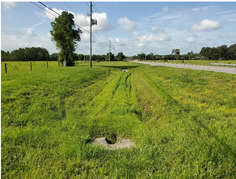
Roadside ditch, facing south
