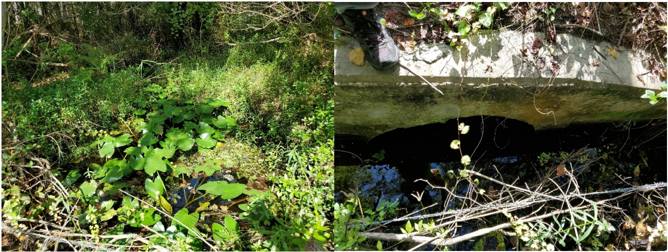
Existing cross drain outlet (west side)
