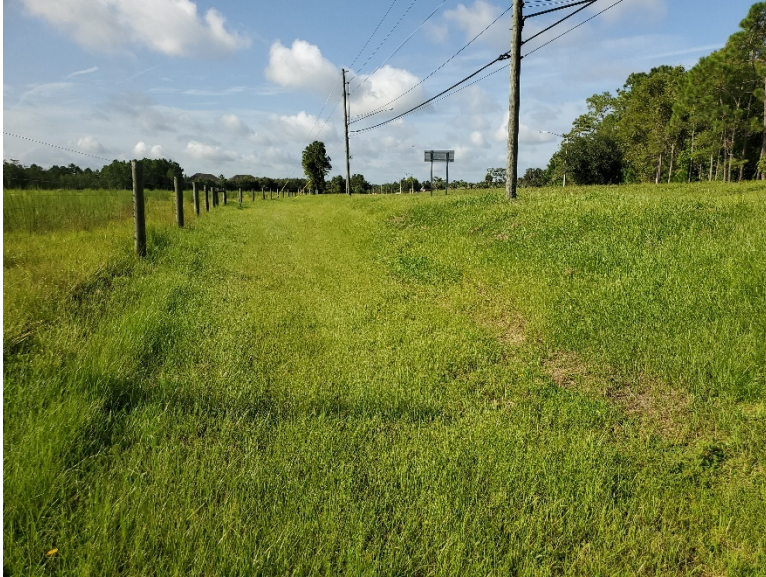
Existing offsite swale, facing south
